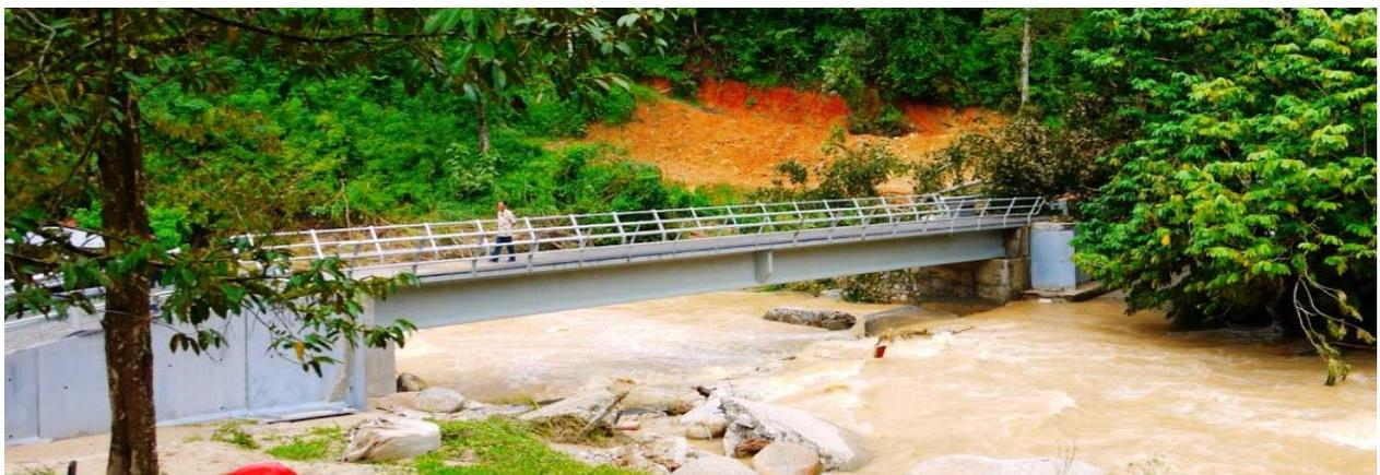
Figure 1 – A 25m single span medium traffic bridge crossing Sungai Itek (Kg. Ulu geroh, Gopeng, Perak) using two pieces of DURA<sup>®</sup> TBG1325.
