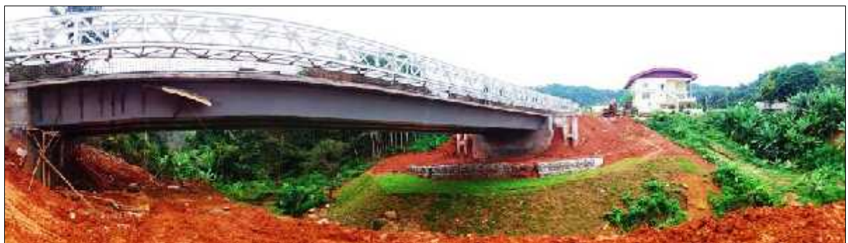
Figure 2 – Newly built single span 50m long Titi Bridge using UBG1750.
