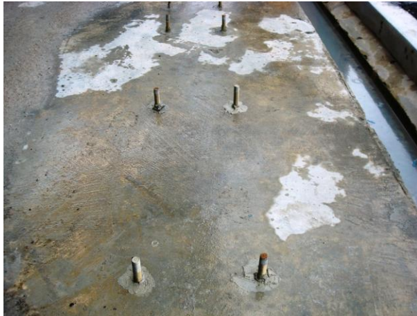
(a) Preparation of Drop-in Anchors on Floor.
