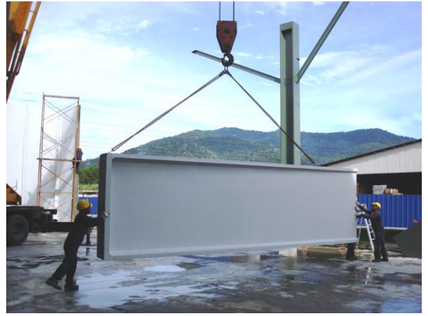
(b) Lifting of Wall WP70/20.
