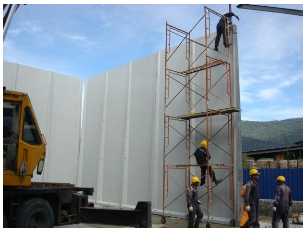
(e) Positioning and Tightening to Adjacent Wall.
