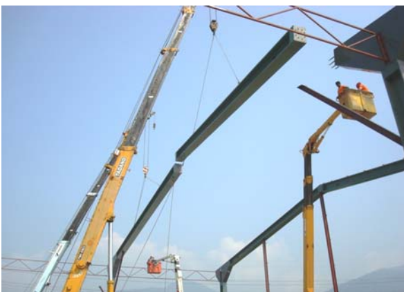
Figure 1 – Dura ® UB-X650 used in portal frame.
